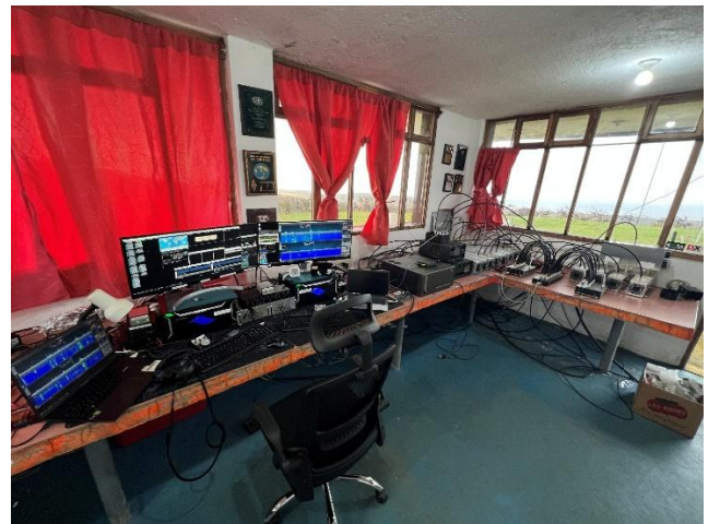
Photo 6 – Overall view of the HD8R shack.
