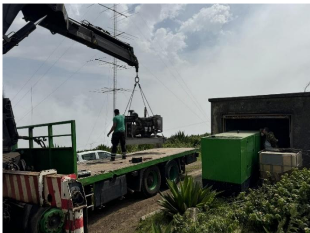
Last minute power generator replacement at D4C
