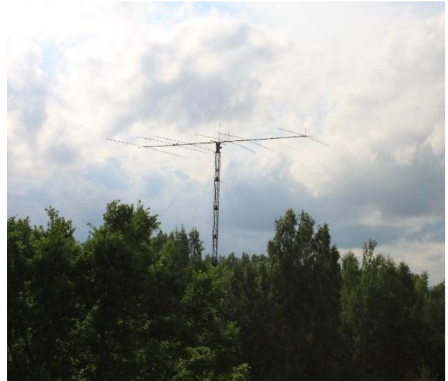
Using this 6-el 20M beauty from ES6Q makes QRP operating more enjoyable for Rein, ES6RW!
