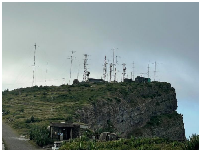
Photo 19 – This is not a military installation; it's the powerhouse station of D4C/D4DX!
